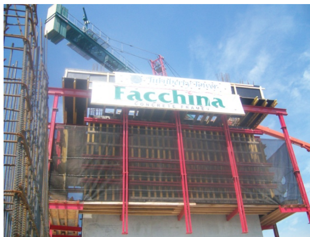
Figure 7.2 – ACS Formwork for Core
